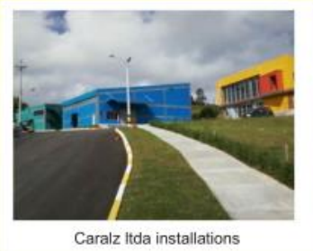
Caralz Ltda installations
