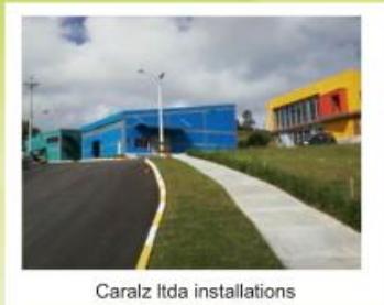
Caralz Ltda installations
