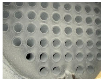
Figure 3-23: Fire-tube boiler (opened) [72]
