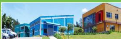
Caralz Ltda installations
