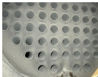
Figure 4-19: Fire-tube boiler (opened) [87]
