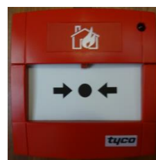
Figure 4-16: Fire alarm [87]
